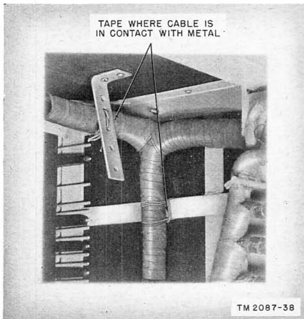
Figure 34. Wire protection; taping to protect insulation.
