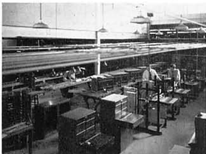
These switchboards are undergoing one of the many stages of routine testing during the process of assembly.
