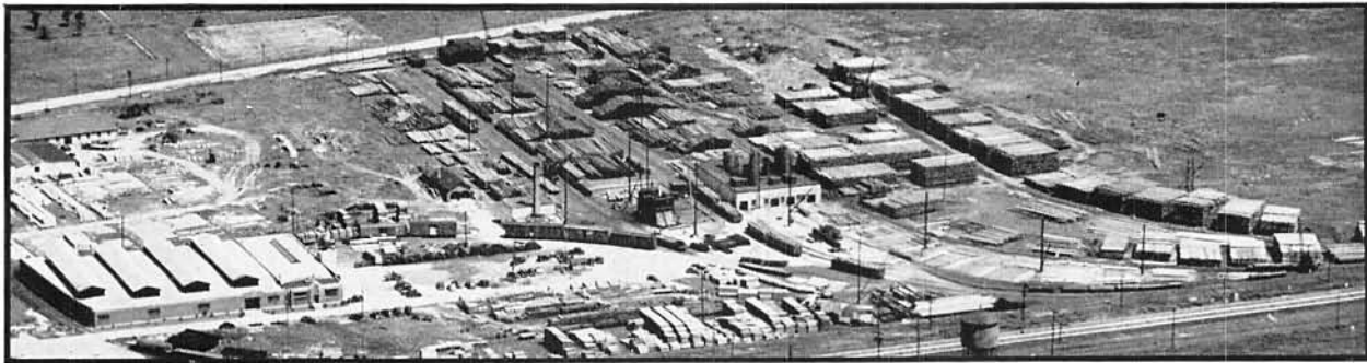
Typical Pole Yard from which Kellogg Poles are Shipped.
