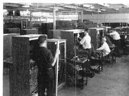
Wiring switchboards, after installing cable and hanging relay gates is a specialty which Kellogg workmen take great pride in doing well.
