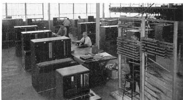
From the iron framework and cabinet shops, these Masterbuilt Switchboards enter the assembly department. Relay-matics are constructed at the right.
