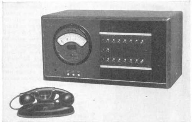
The Kellogg Senior Test Cabinet is designed as an aid to the wire chief in the average common battery exchange where proper maintenance of lines and equipment is of first importance. With this equipment, line, instrument or exchange troubles may be quickly and easily located. The Senior Cabinet is larger, more completely equipped, and more flexible than the Junior model.
