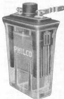
**Flote' Type** — Philco batteries are of the Faure or pasted plate type and feature Flote' special grids and plate construction. The active material is firmly pressed into the plate and locked in place, by virtue of crossing grid members on opposite plate surfaces.
