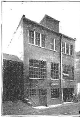
Rear View Columbus Warehouse Showing Trackage Facilities
