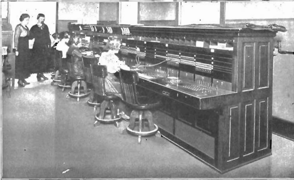
Eight-Position Kellogg Toll Switchboard at Eldorado, Kansas
