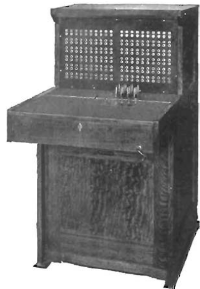
Sixty line floor type toll test panel, 4 jacks per line
