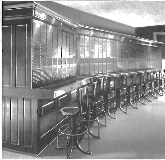
New Service Board Installed at Freeport, Ill.
