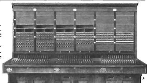
A 300-Line Universal Switchboard
