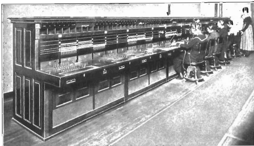
12 Pos. Kellogg Toll Switchboard at Ada, Oklahoma
