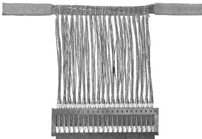
Flat Cable Soldered to Spring Jack.
