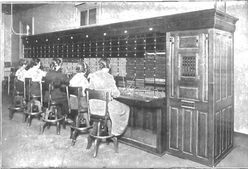
A Service Switchboard of 2,400 Lines Installed at Jacksonville, Illinois
