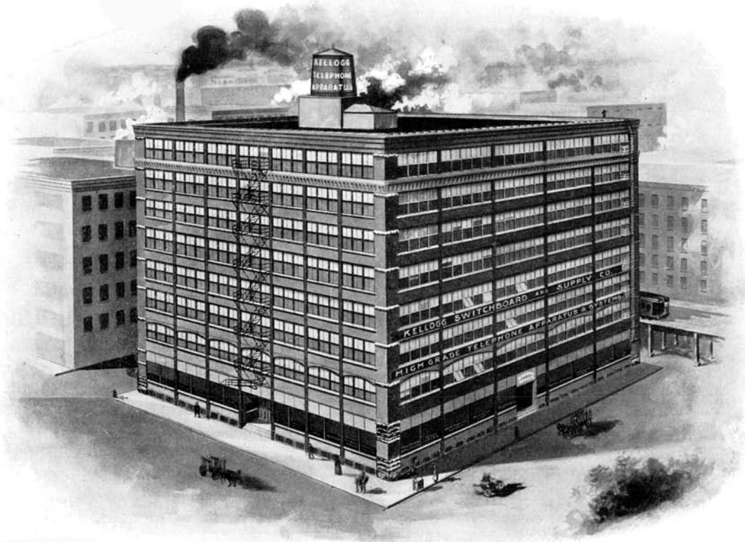
MAIN FACTORY AND GENERAL OFFICE
