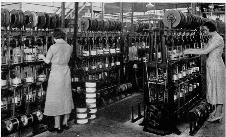
90 MILES A DAY! This is the kind of speed at which these machines insulate wire and tinsel. Each machine of this group applies up to 3 coverings of silk or cotton to 6 different conductors AT THE SAME TIME! Only purified silk and long-fibre cotton of the highest grade are used.
